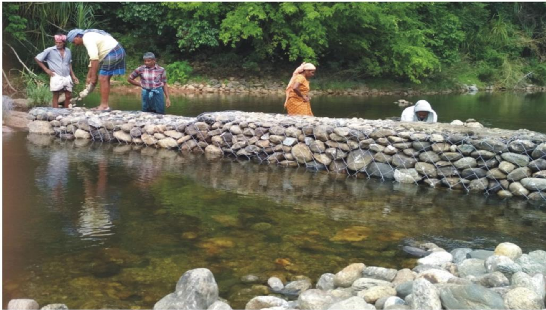
Construction of Gabion checkdam-Kunthipuzha Thachampara Grama Panchayat in Mannarkkad block Persondays-332, Expenditure Rs.125000
